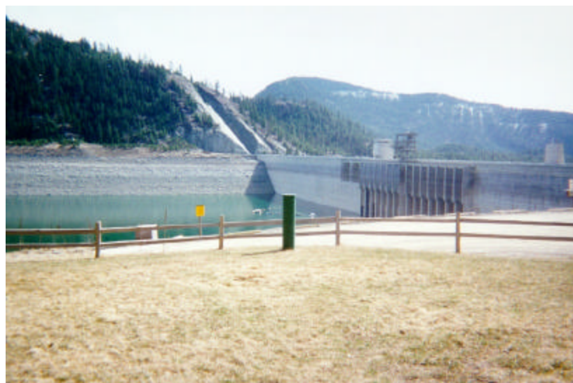
Figure C-4. Reference Station (R2), Libby Dam.
