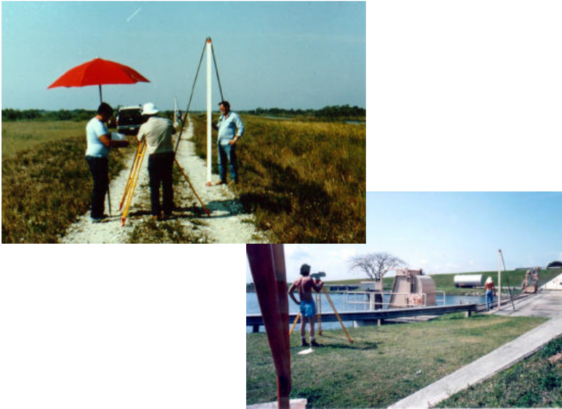
Figure 6-1. Precise leveling runs on levee in Everglades and gate structure. Parallel plate micrometer level with invar rods. (Jacksonville District)
