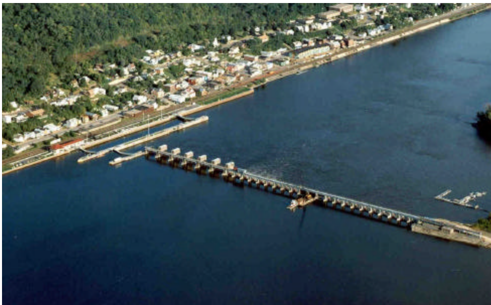
Figure B-2. Aerial View of Lock and Dam No. 4, Alma, WI.
